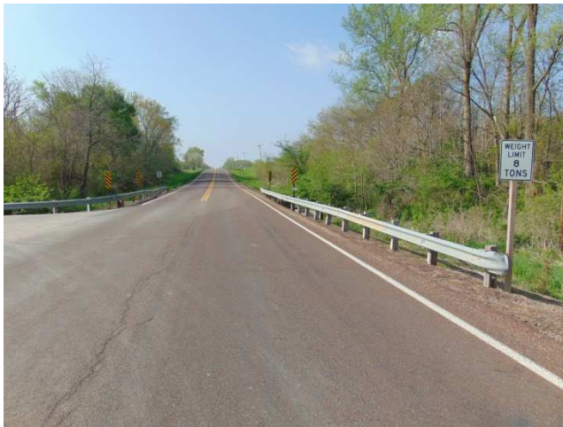
Looking south across the bridge
