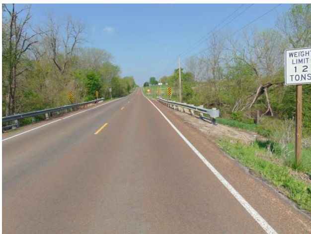
Looking west across the bridge
