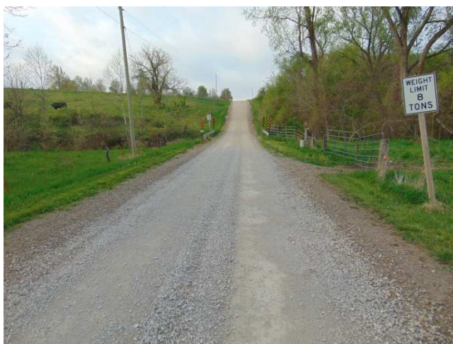
Looking south across the bridge
