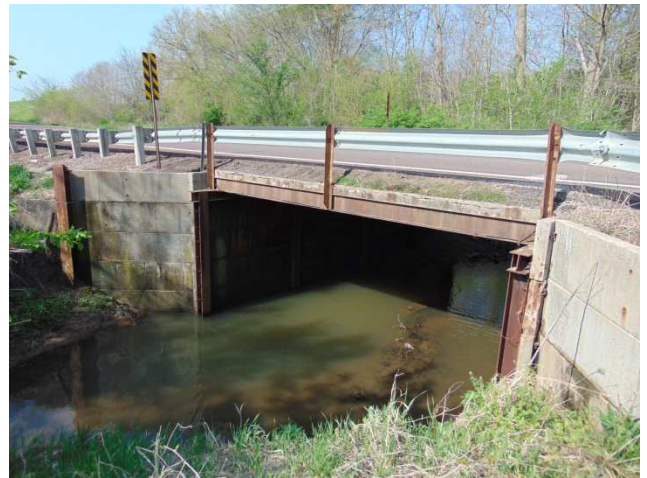
Elevation view looking southwest
