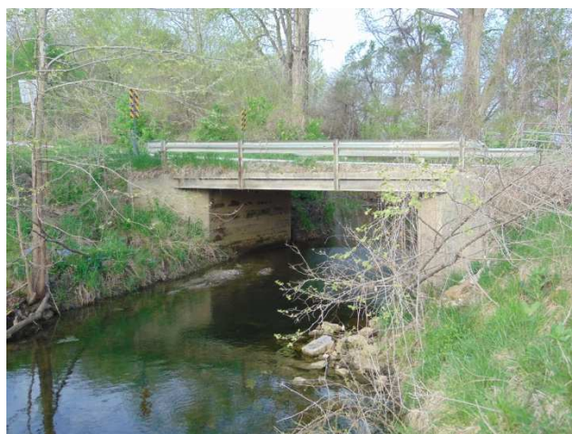
Elevation view looking west
