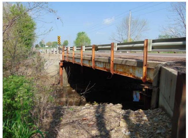
Elevation view looking northwest
