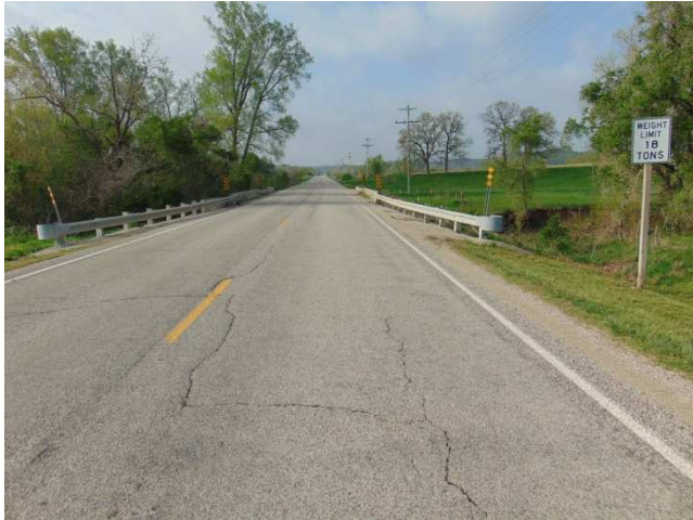
Looking south across the bridge
