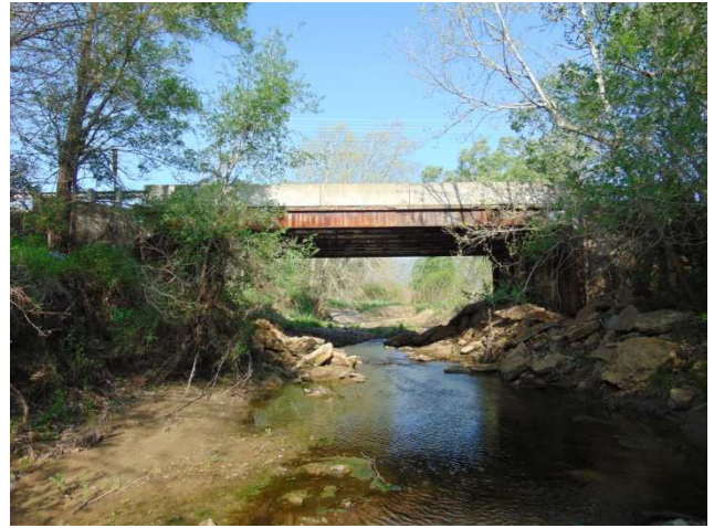
Elevation view looking west
