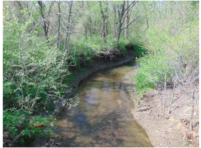
Looking downstream from bridge
